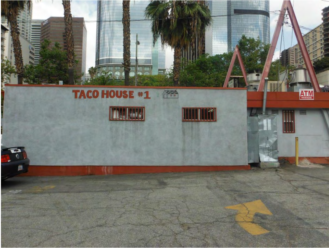
Photograph 11: Looking northwest at rear of Taco House.
