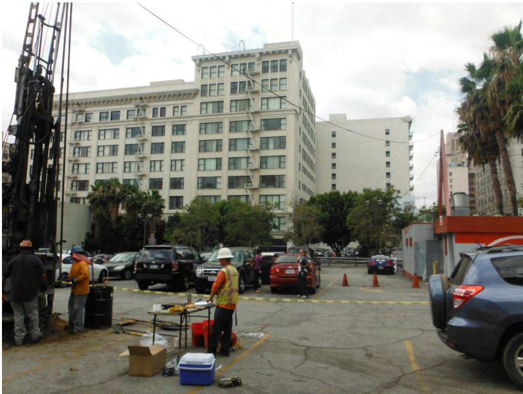
Photograph 8: View from Property looking southwest at southwest adjacent properties (Junipero Serra office building and parking lot).
