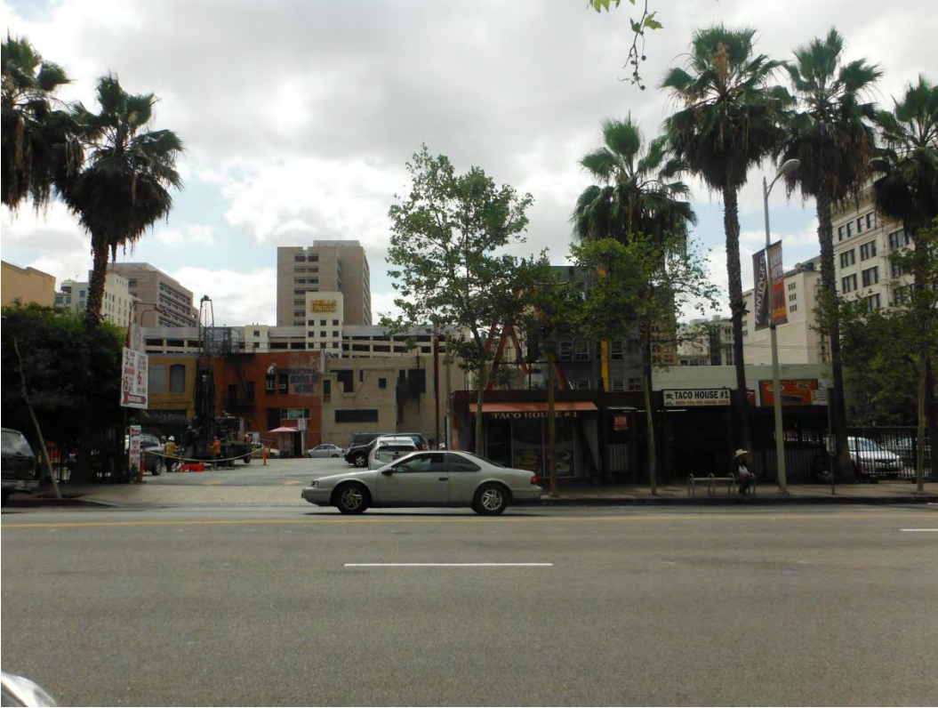
Photograph 1: View of Property looking southeast (across South Hill Street).
